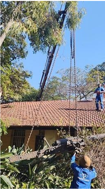
Prepping to rig out & over
